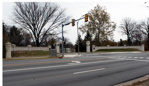
NIU Main Entrance on Castle Drive
