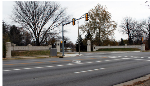
NIU Main Entrance on Castle Drive
